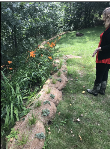
Stormwater Control Berm
